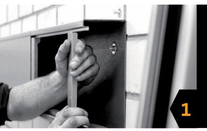
The installation engineer can choose between three different dimensions for various cable volumes. The ducts are delivered in lengths of 2 metres and are thus also suitable for simple, rapid section mounting.
