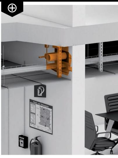
A sensitive area which is frequently forgotten: The underfloor cables. But the area under the system floor must also be well insulated. In server rooms with system floors, dust and fibre-free systems are suitable, as great emphasis is placed on cleanliness.
