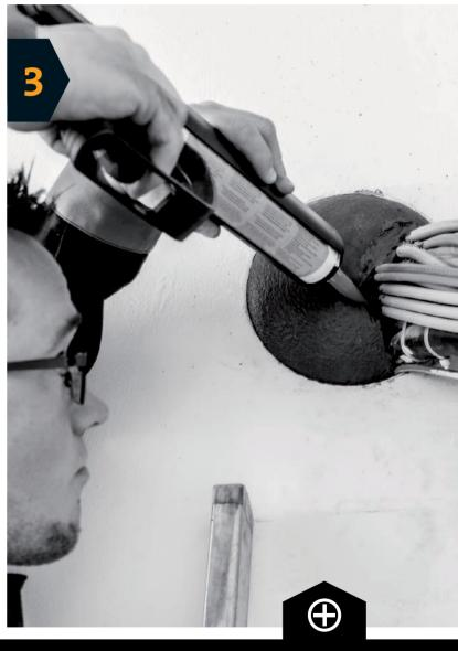
The installation engineer cuts the plugs according to the cable assignment. Then they are pressed into the wall opening quickly and cleanly on both sides - without dust or fibres. Installation must always take place according to the approval.
