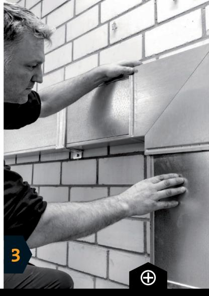
With the PYROLINE® Rapid duct system, the electrician can simply snap on the lid after installing the cables - without the use of screws or tools. Connectors provide smoke closure: The closing contour between the lid and base provides effective sealing. For the fire protection ducts, many different fittings are available for horizontal or vertical changes of direction. Here, the installation engineer is mounting a flat angle after having installed the cables beforehand.
