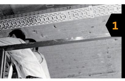
The installation engineer always selects the material of the cable trays according to the existing regulations. In our road tunnel, section mounting takes place with a special tunnel clamp made of rustproof steel. Alternatively, many other mounting versions are also available, e.g. with suspended supports and brackets.
