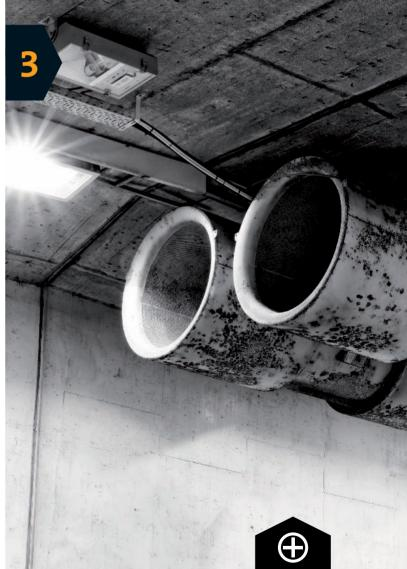
Junction boxes, which protect the cables against external influences such as dust and water, are used to branch and extend the cables. Here, the OBO FireBox is installed directly on the tray. Alternatively, mounting on the wall or ceiling is also possible. A fireproof connection of wires is ensured through ceramic terminals.
